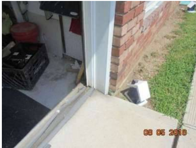
Photo 30-2 No damage noted on the exterior
