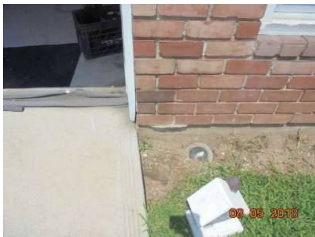
Photo X-3 Termite bait system.
