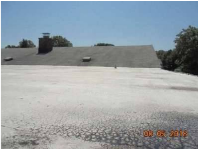
Photo X-1 View of roof. No recommendations at this time.
