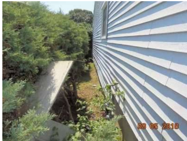
Photo 3-2 East side of house
